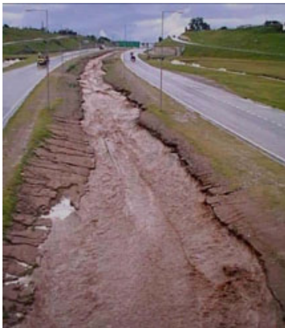
Figure 6.30. State of the central canal of the north-east section during the storm of December 2003.
