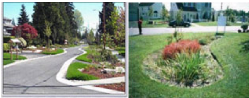
Figure 3.24. The photo (left) shows a street without a kerb allowing part of the runoff to infiltrate into the grass alongside. The photo (right) depicts an infiltration area in a flower bed.
