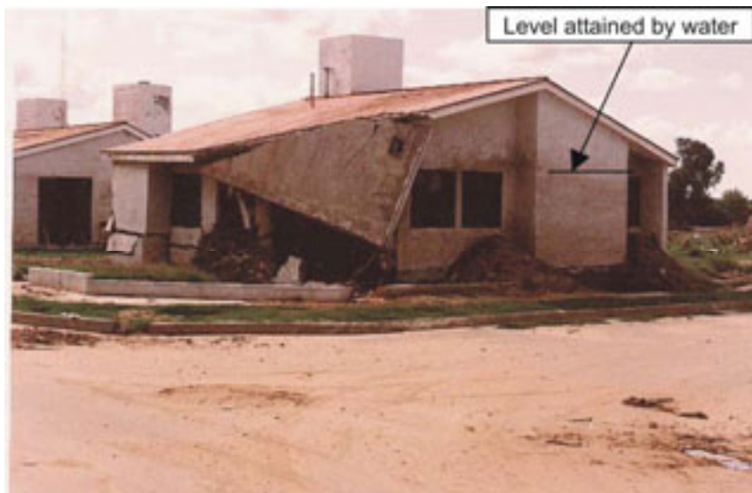
Figure 6.44. Damage to dwellings in a district of San Carlos Minas, Argentina. Flooding, January 1992.
