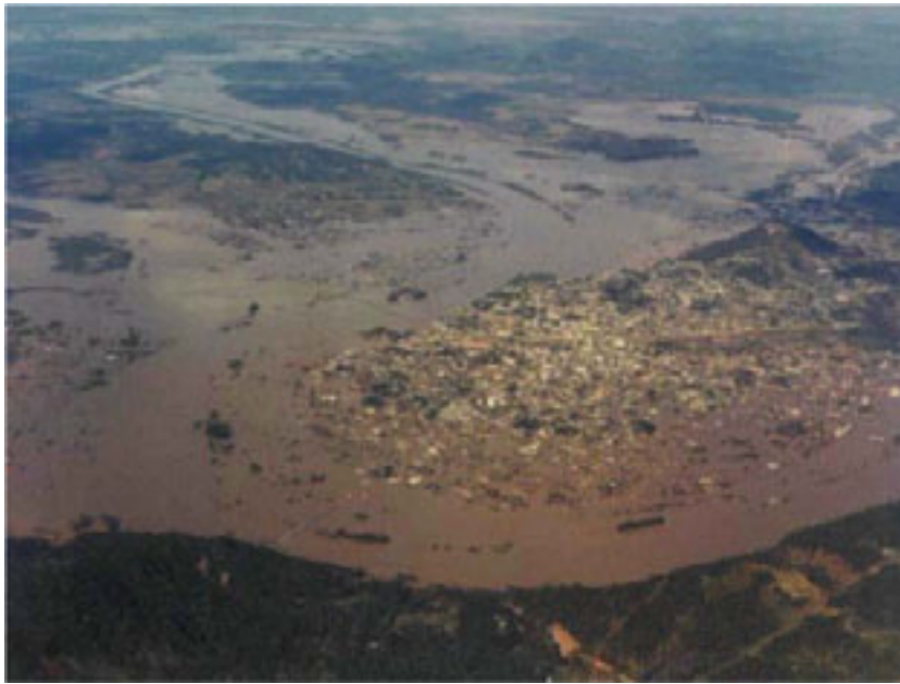
Figure 6.3. União da Vitória and Porto União during the 1983 flood
