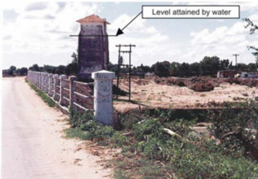
Figure 6.43. Area immediately upstream of the bridge. Event of January 1992 at San Carlos Minas, Argentina (Source: Barbeito et al. , 2004).
