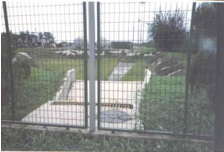
Figure 6.22. Detention basin built for a private project. Córdoba, Argentina (Source: Toya et al. , 2003).
