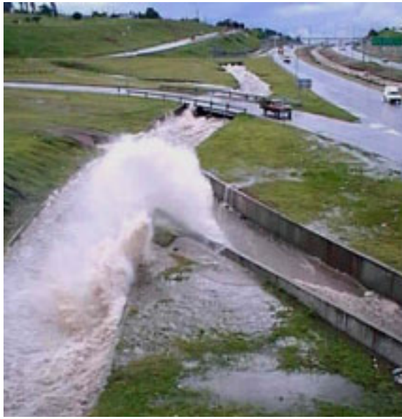
Figure 6.29. The inner canal during the storm of December 2003. Note the effect of the poor hydraulic design of the transition.
