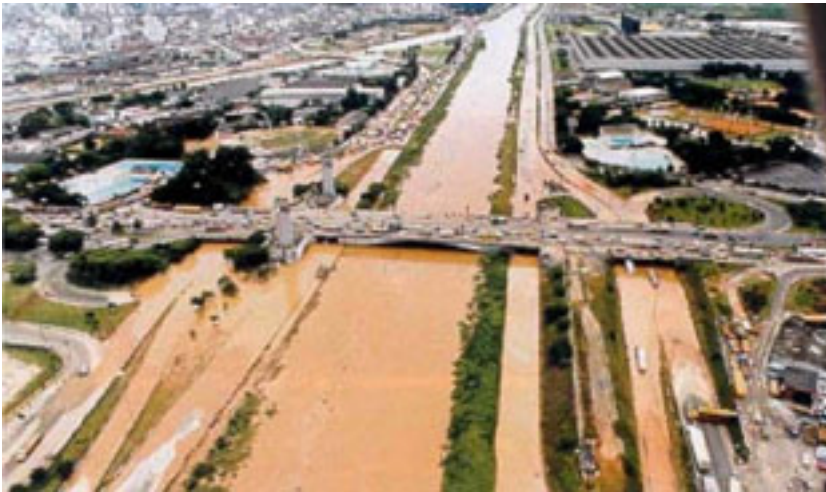
Figure 3.15. Flooding of the river Tietê at the Bandeiras bridge as a result of urbanization of the city of São Paulo.
