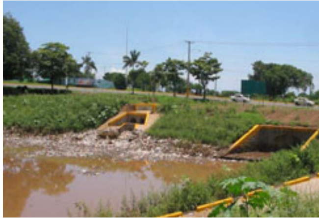
Figure 6.64. Concentration of urban refuse in the Los Gauchos Tiscapa microdam, opened in 2005. City of Managua.
