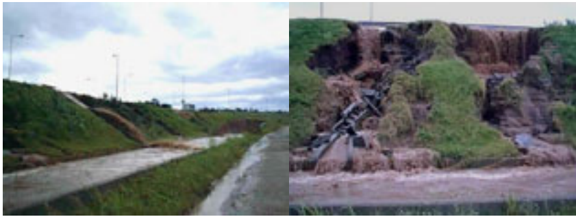
Figure 6.27. Damage to the outer canal during the storm of December 2003. Situation before and after the peak of the flood.
