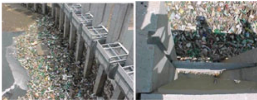
Figure 3.8. Refuse accumulating in drainage (São Paulo - Brazil)
