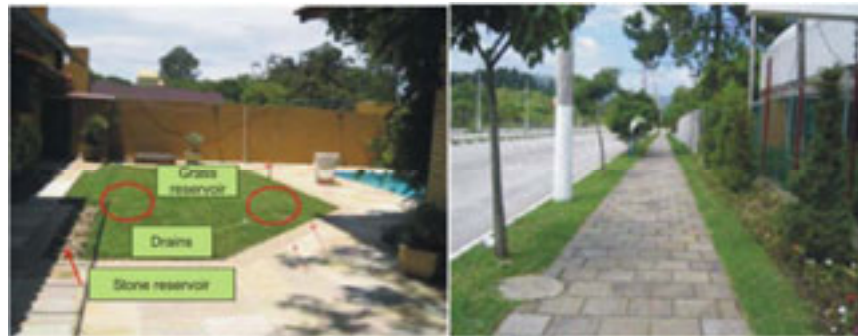
Figure 3.22. Use of systems for retaining water from impervious areas (a) the left-hand photo shows drainage from paved areas onto grass and from roofs into gravel reservoirs; (b) paths with grass alongside to increase infiltration.
