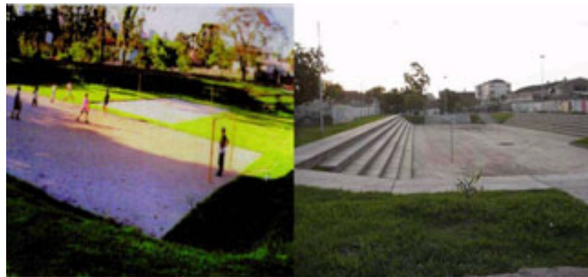
Figure 3.35. Detention basins used as sports fields in Curitiba (left) and Porto Alegre (right)
