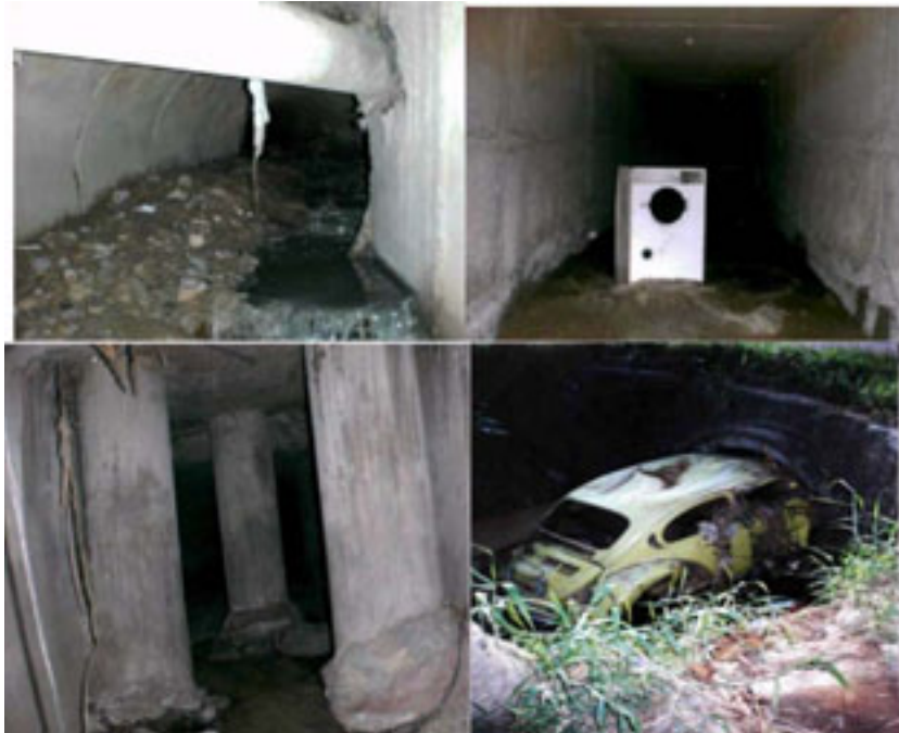
Figure 3.7. Obstructions and refuse in the drainage (Belo Horizonte and São Paulo – cities in Brazil)
