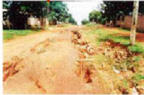
Figure 3.5. Erosion of unprotected urban area (Campana, 2004)
