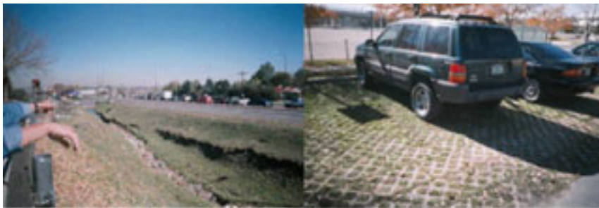
Figure 3.23. The photos show (left) an example of infiltration trenches and (right) pervious paving with perforated blocks for car parking
